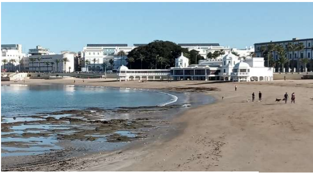
Control on the beach-side corner of the raised building
